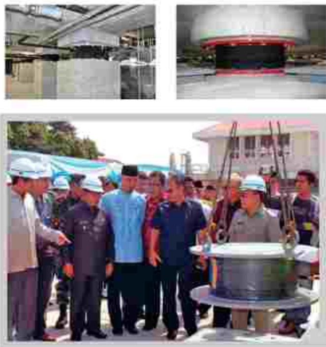
Figure 4.18 Detailed of Seismic Isolation on Building
