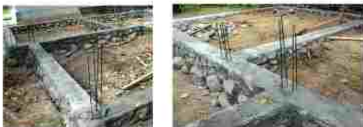
Figure 4.11. River Stone Foundation
