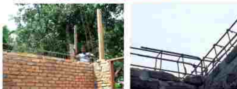
Figure 4.15 Peripheral Beams and Ring Balk
